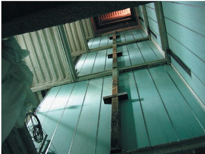
important wall assemblies in a building. Vertical chases and mechanical enclosures keep vital communication, power, water, fresh air and exhaust systems intact when a fire occurs.
