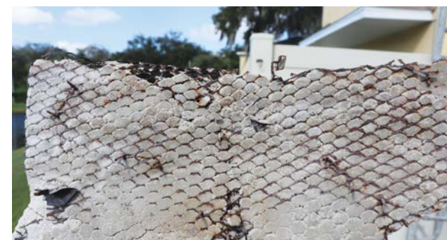
Corrosion can stay on a wall for years and then "give away" from a storm or wind event.
