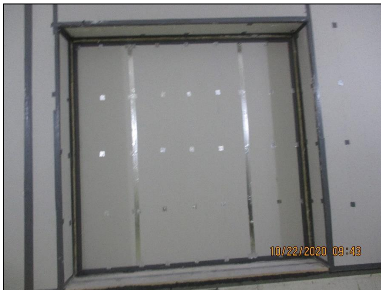
Photo No. 2 Source Room View of Installed Specimen
