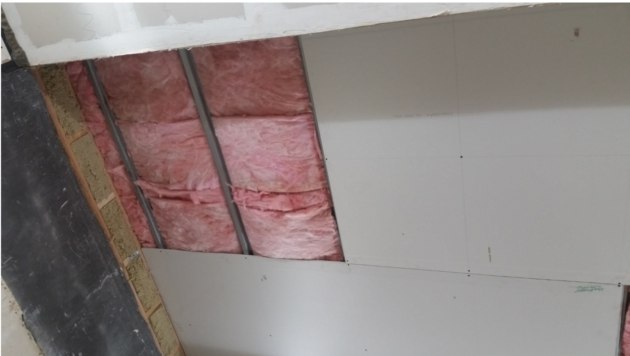
Figure 8 – First layer of gypsum board partially installed to furring channel
