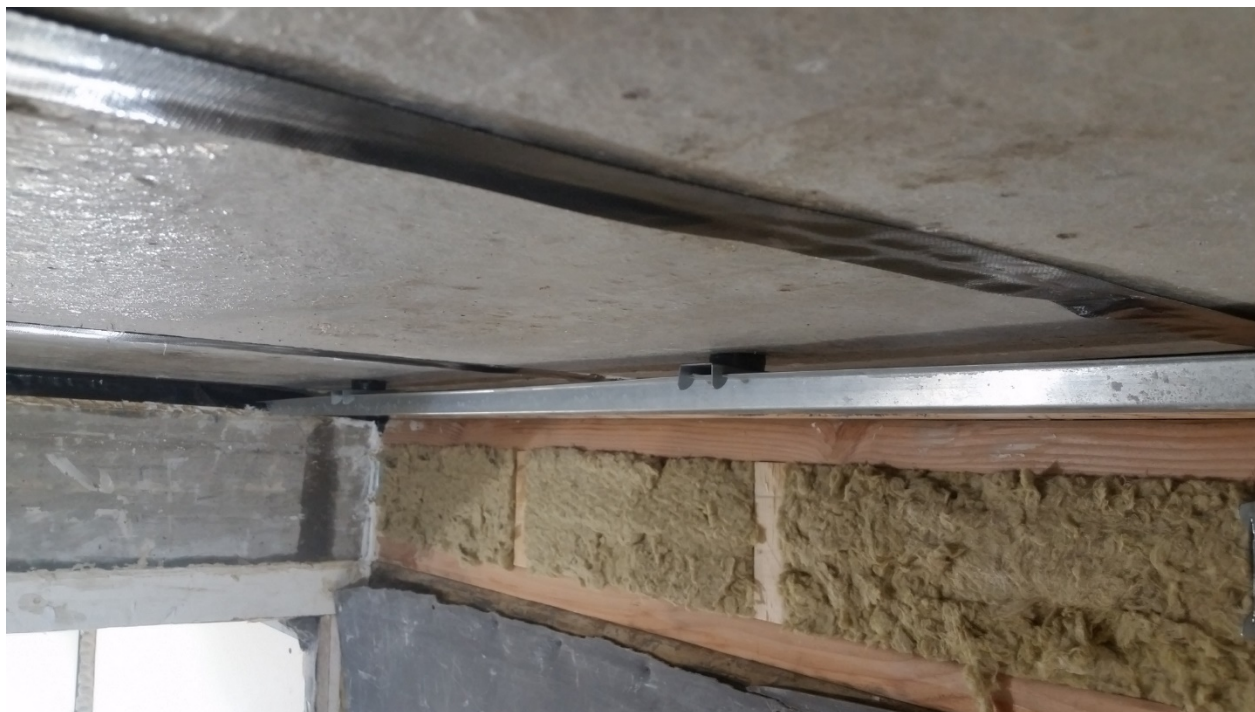
Figure 6 – Furring channel being installed to isolating clips
