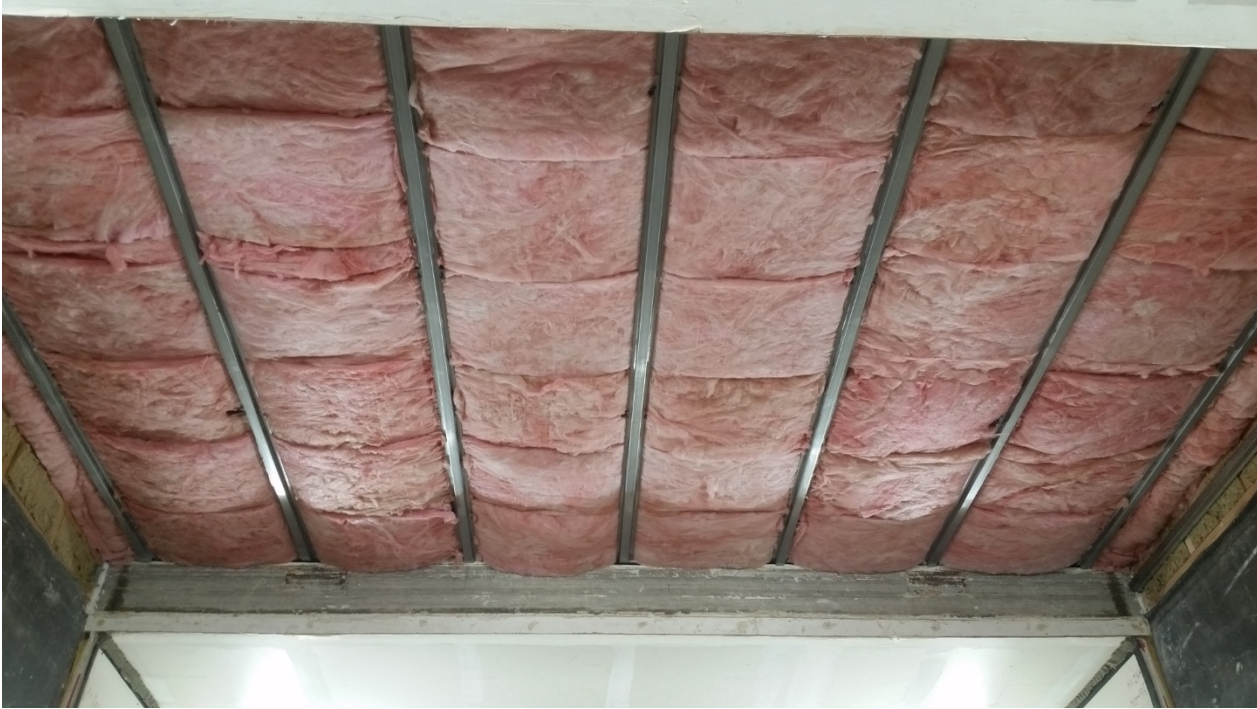
Figure 7 – Furring channel and insulation installed below slabs
