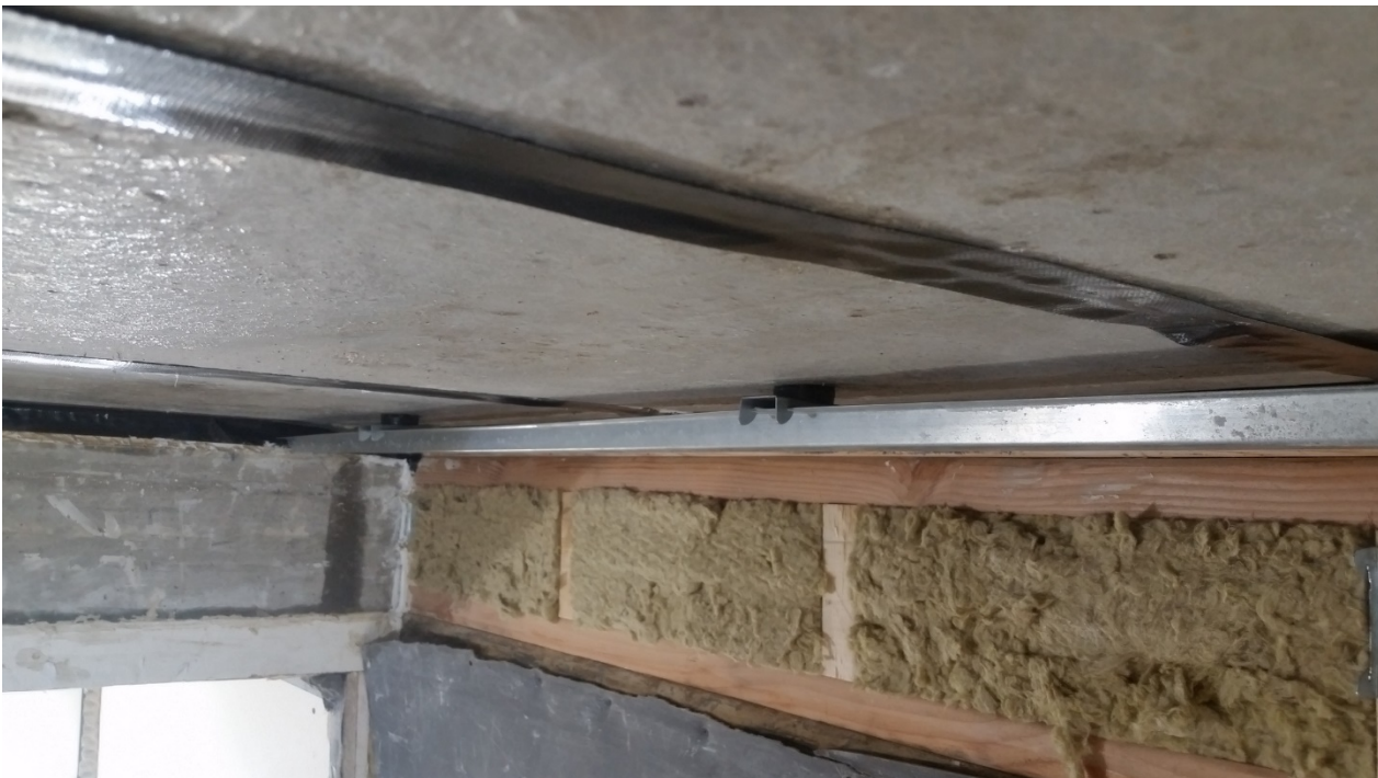
Figure 6 – Furring channel being installed to isolating clips
